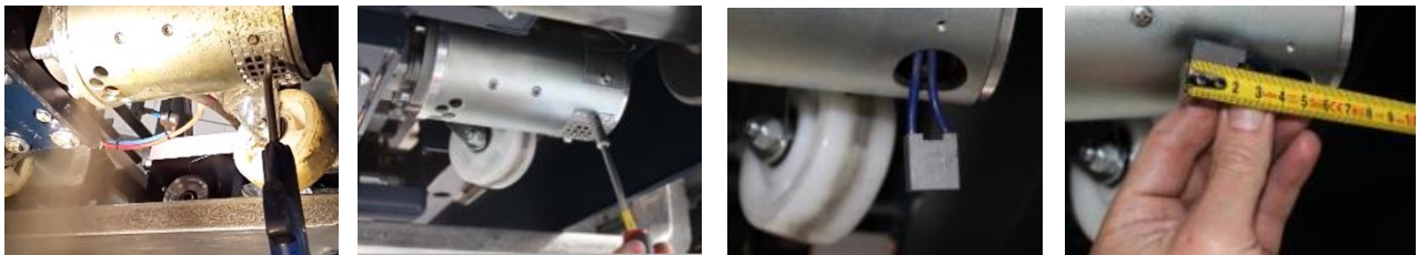
Figure 9.4; Inspecting carbon brushes in the motor
