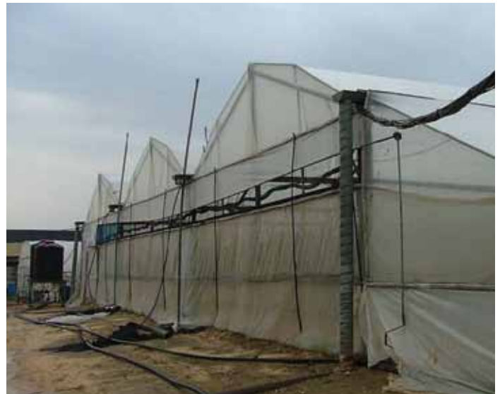
Tomato greenhouse, 501 sprinklers on the roof along the gutters
