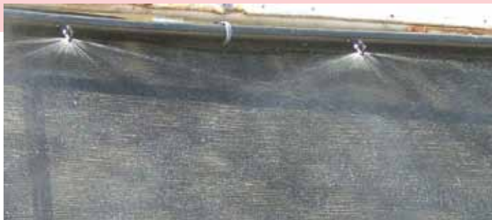
Modular half-circle sprayer 100 l/h mounted every 1.0 m
